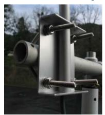
• Tighten nuts, keeping sensor level.
